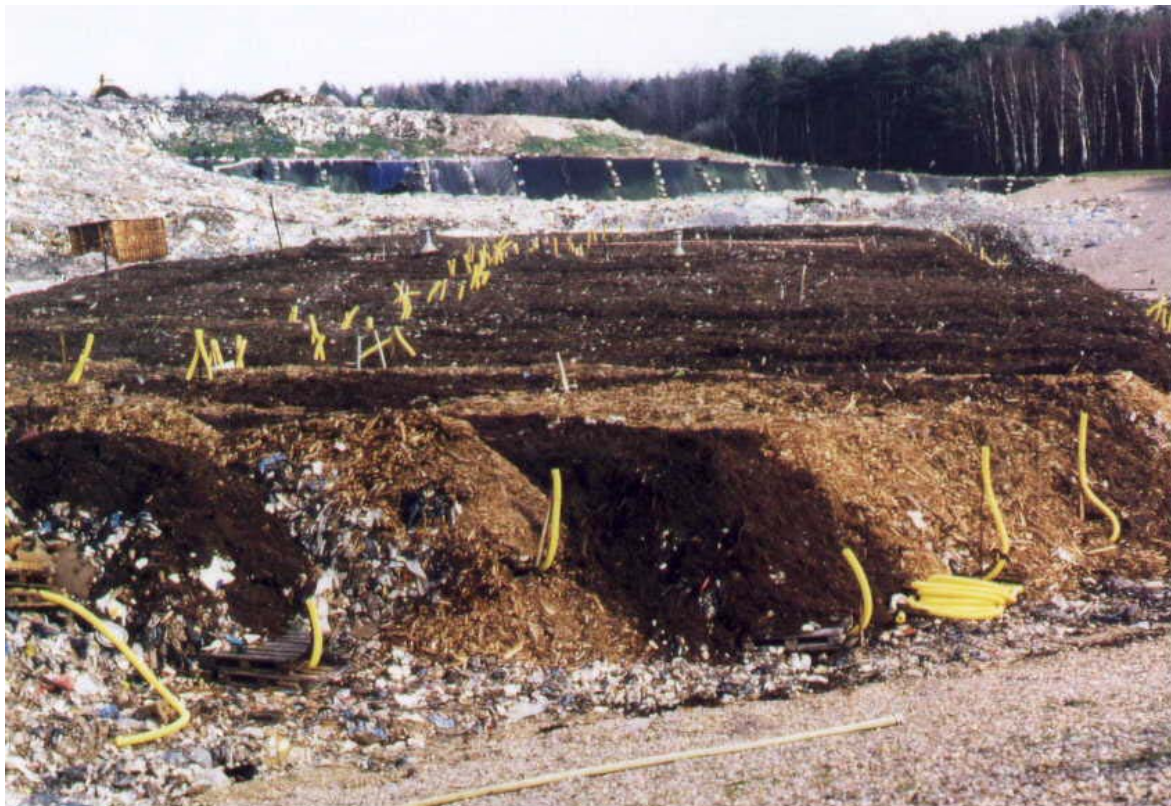
Figure 5: Chimney-effect system at Meisenheim landfill (Germany)
