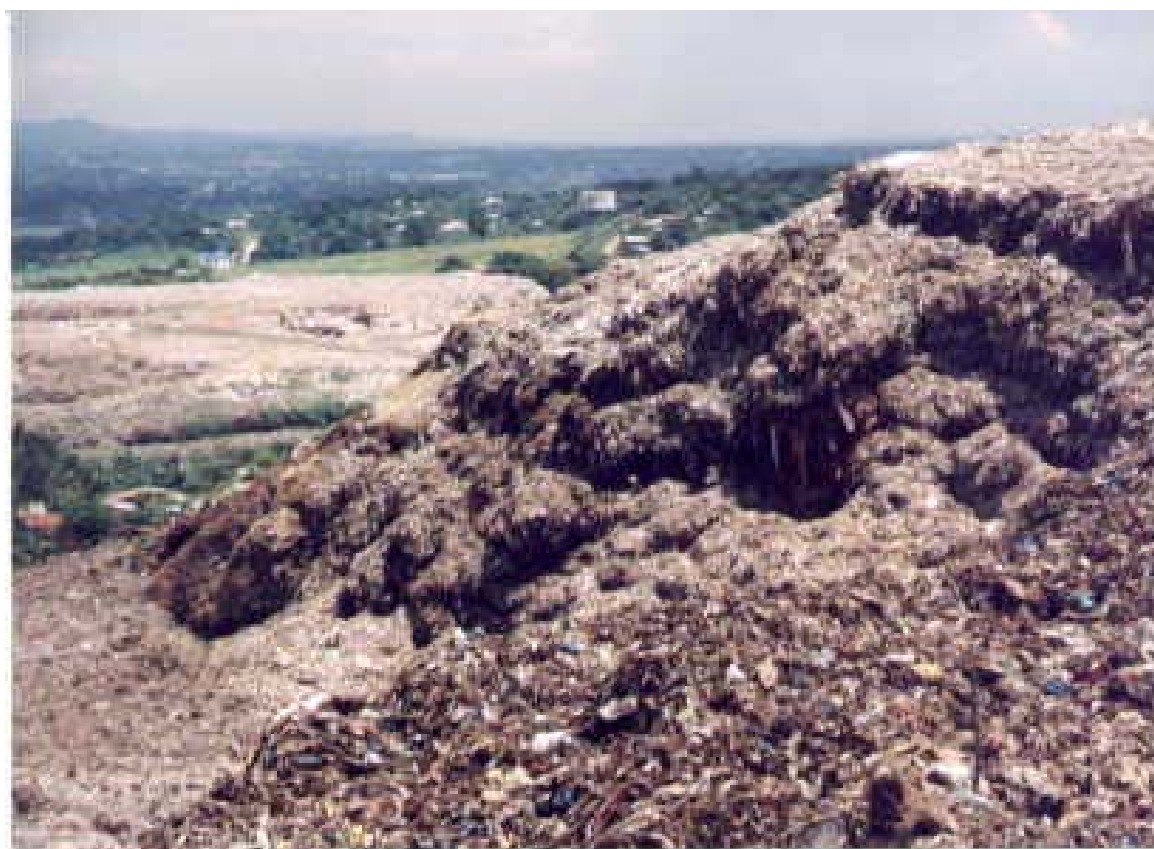
Figure 3: Broken slope at Payatas dumpsite – August 2000
