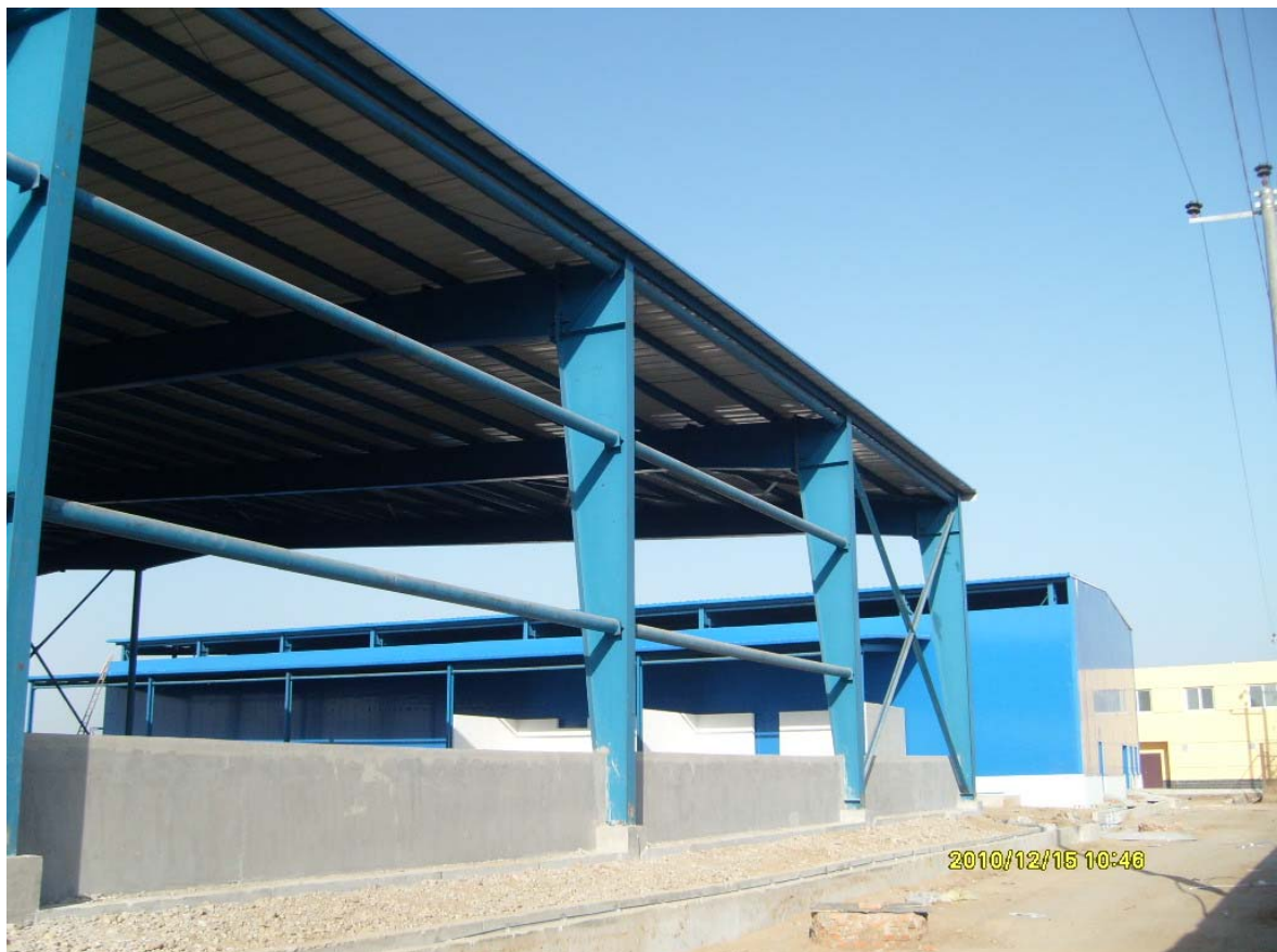
Figure 9: Facility compounds - biological treatment (in front), delivery (background)
