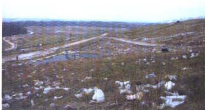
The eastern slope of the Ihlenberg landfill, where the cessation of waste dumping had caused a depression in the landfill's geometry
