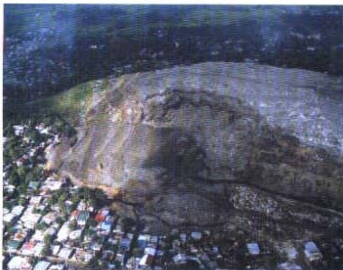
ABOVE A landfill failure in Payatas, the Philippines, killed more than 200 people. Waste and debris completely covered an area of around 30,000 m 2 in front of the toe of the slope. BELOW The collapsed slope of the Payatas landslide four weeks after the event. FACING PAGE Landfill failure in Athens, Greece. In this landslide, about 800,000 m 3 of waste moved, leaving a 300- to 400-metre-wide gap in the slope behind.
