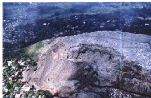
Photo 1 : Rainfall-induced failure of municipal waste at Payatas, the Philippines (by R.Orense).
