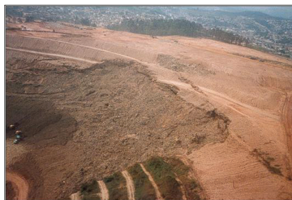
Figure 7: Slope failure of Bandeirantes landfill, Sao Paulo, Brazil in 1991 (Borgatto, 2007)
