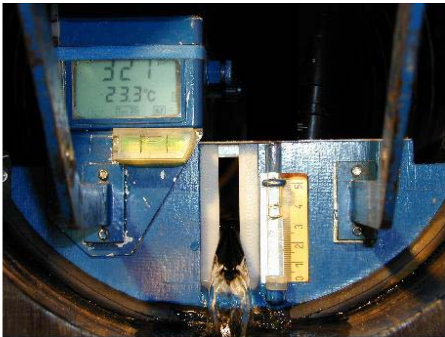
Figure 9: camera view on the operating weir and spillway inside the pipe
